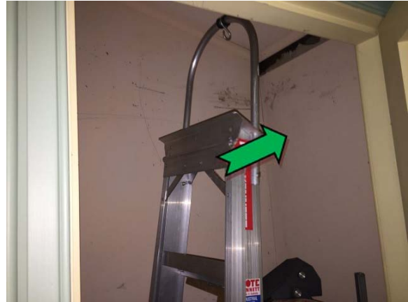
Photo 2. Interior, southern elevation, east cupboard, lining – non asbestos-containing fibre cement sheeting.
