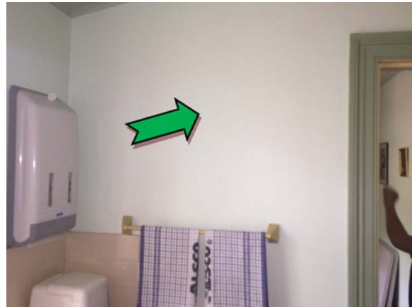
Photo 4. Interior, kitchen, western wall – assumed non asbestos-containing fibre cement sheeting.
